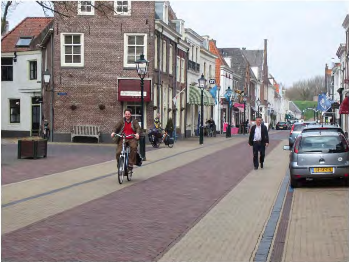
Figure 6-1: Mixed traffic road using colour for visual narrowing
