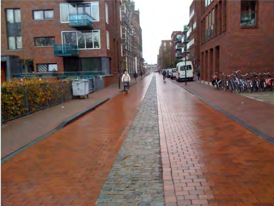
Figure 6-2: Mixed traffic environment using colour and texture to narrow and separate direction
