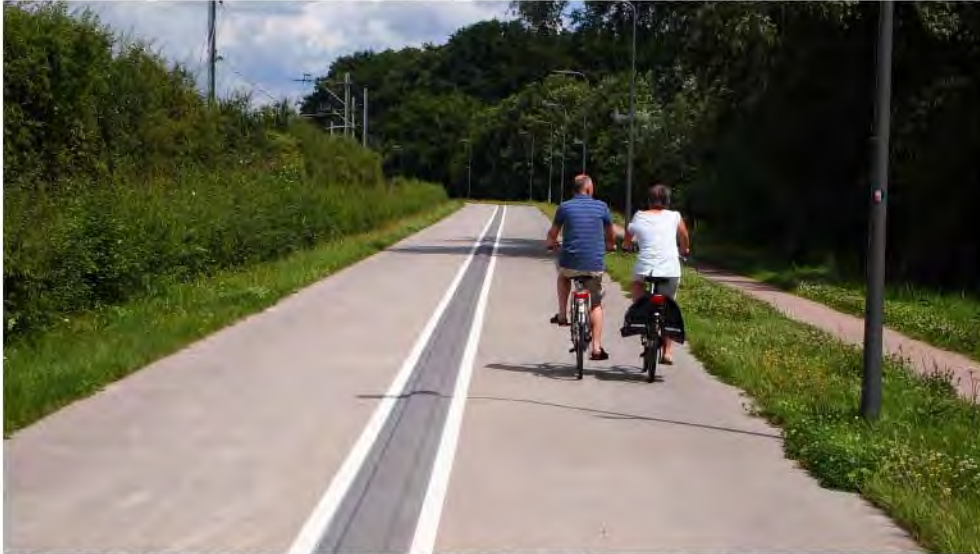
Figure 6-4: Cycle path with directional separation to improve comfort
